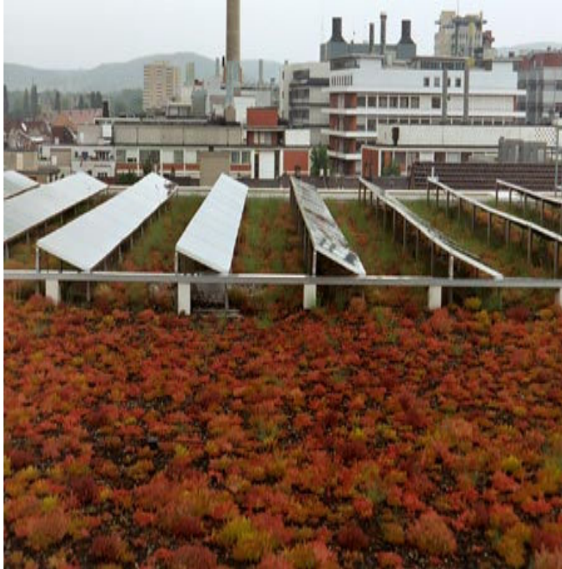
Brown roof with photo voltaic panels
