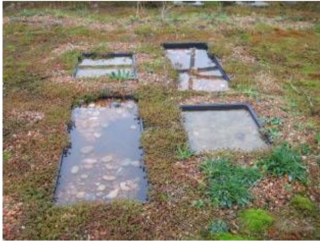
Green roof with water feature
